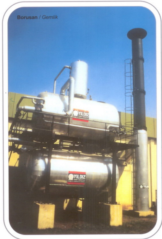
25 m 3 /h DEGAZÖR ve BESİ SİSTEMİ 25 m 3 /h DEAERATOR and FEEDING SYSTEM
